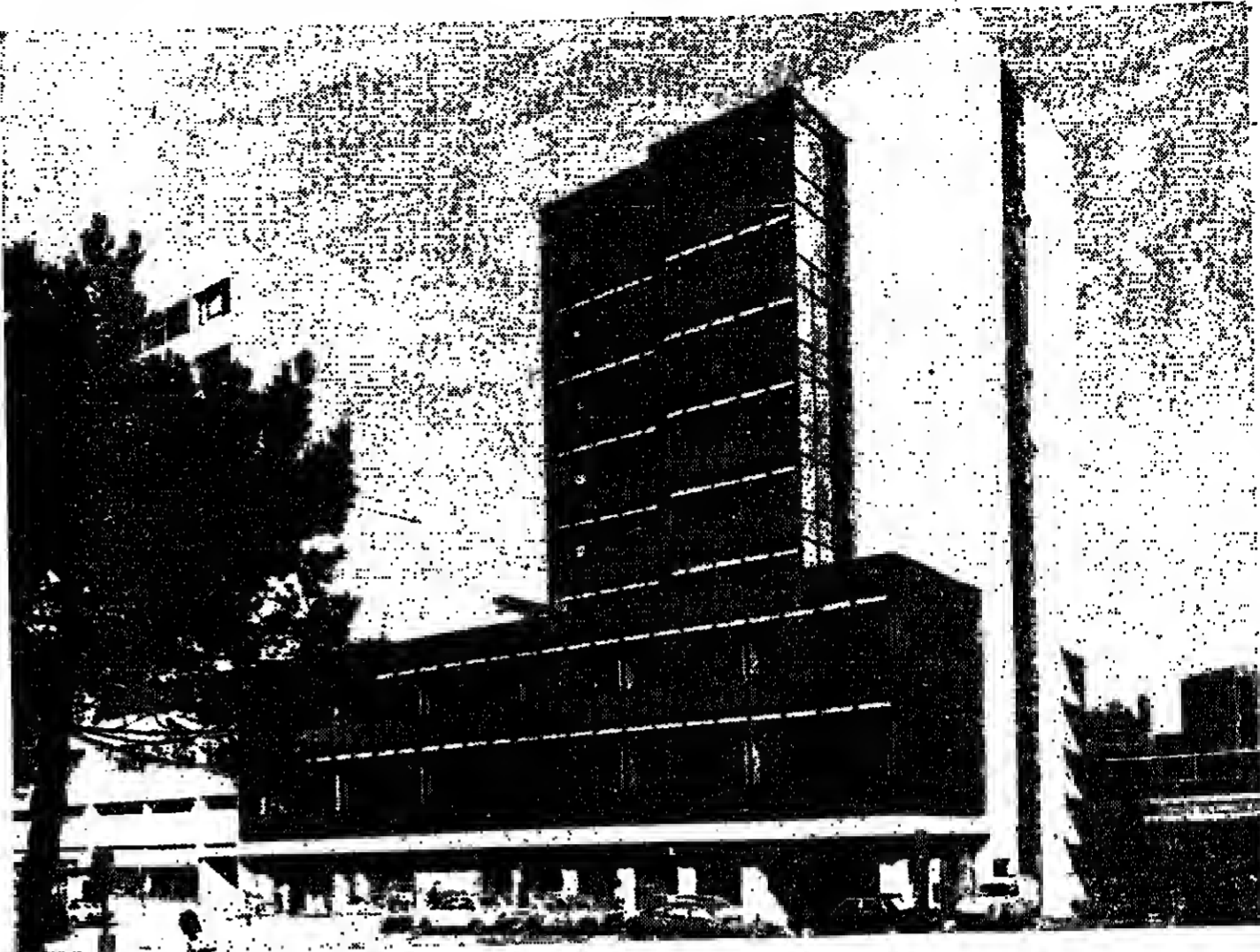
The 41,000 sq ft of air-conditioned office space in Heron House, Bournemouth, is available for letting through agents Jones, Lang, Wootton and Goadsby & Harding. The ground floor plus basement have already been let to National Westminster Bank.
